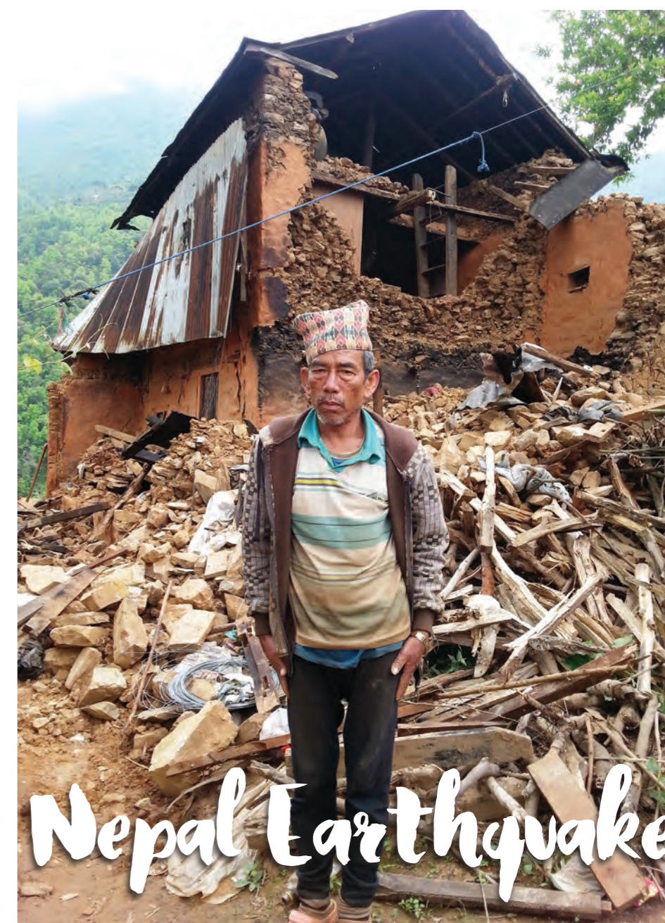
Shyam Tamang stands outside his collapsed house destroyed by the earthquake on 25 April 2015. Photo taken in May when TLM Nepal needs assessment team visited Dhading district, north-west of Kathmandu.
